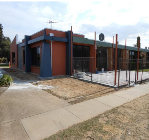
The pergola roof has since been completed
